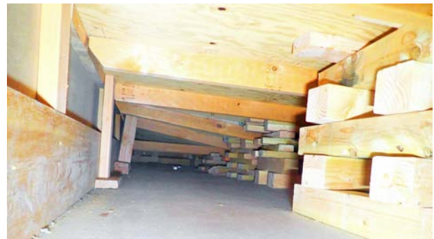
Timber shoring in place underneath the display
