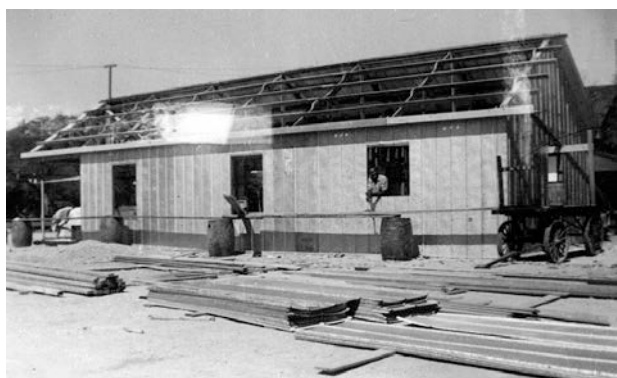
Crowbar under construction
