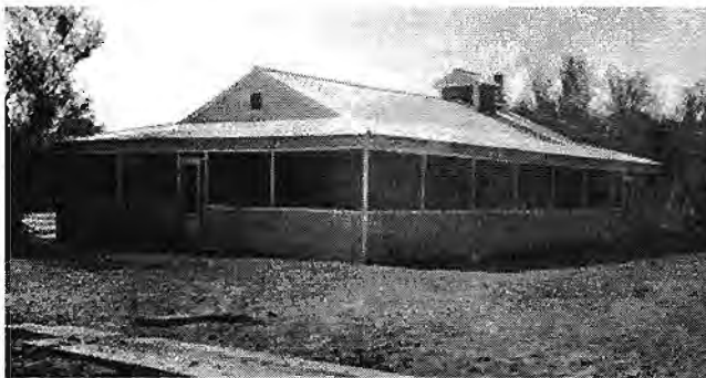
Adobe building completed.
